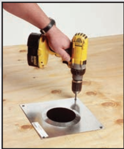
Mount SureGrip support plate.
