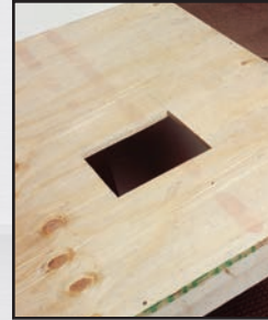
Cut the hole.
