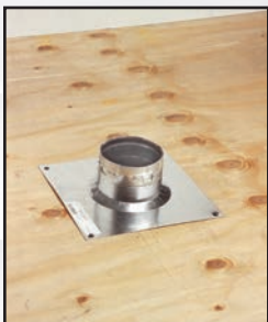
Push pipe through vent support.
